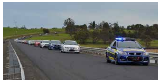
Route 69 Cruise over the Blue Rock Dam wall
