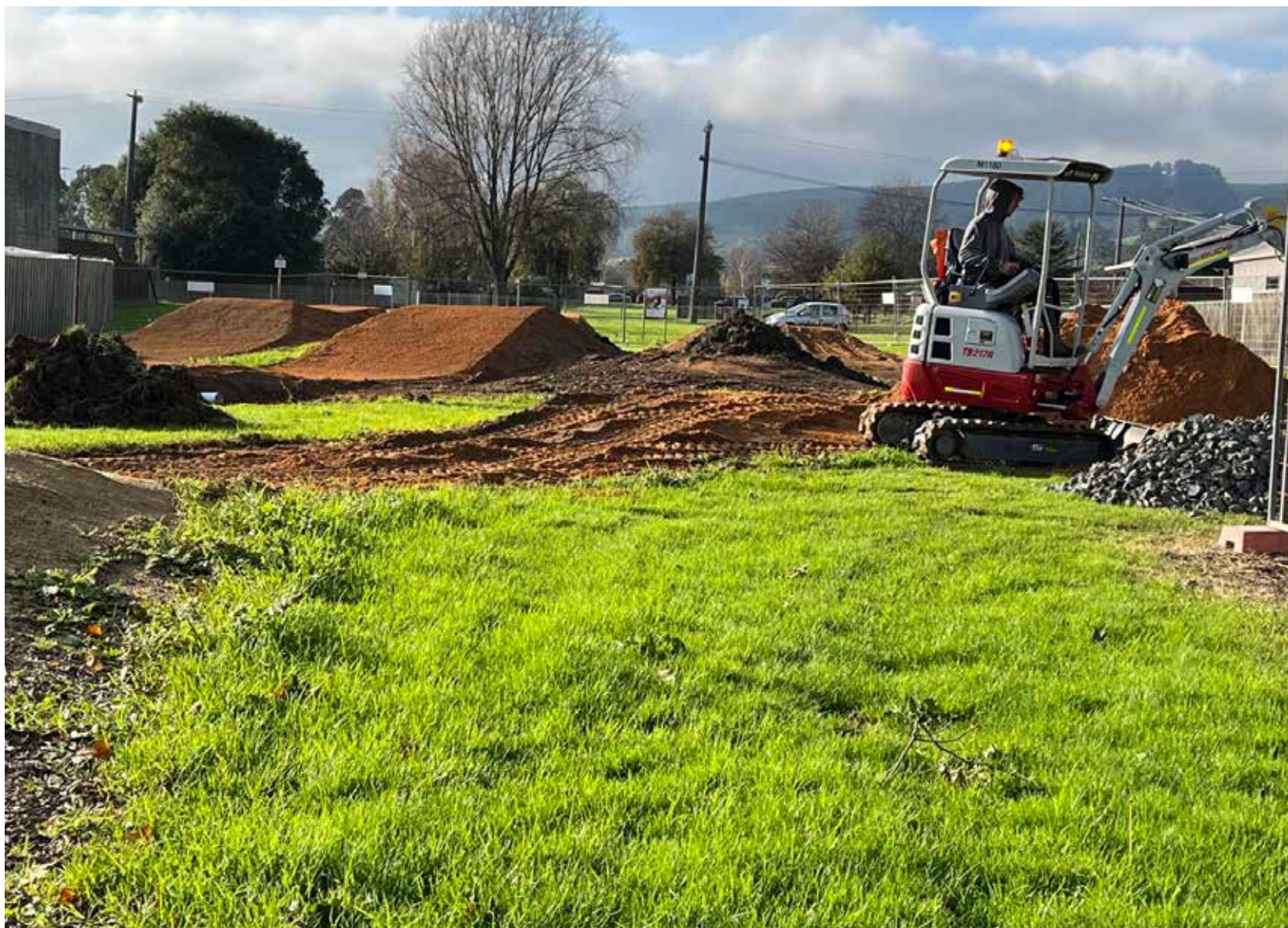
Work underway at Trafalgar's BMX Park
