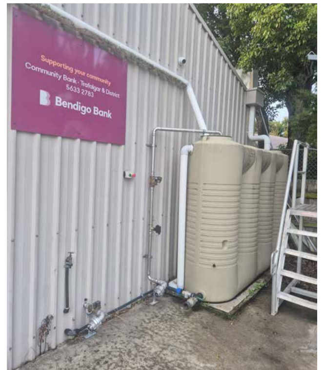
The grey water recycling system funded in part by Community Bank Trafalgar and District, and brigade funds collected as donations.
