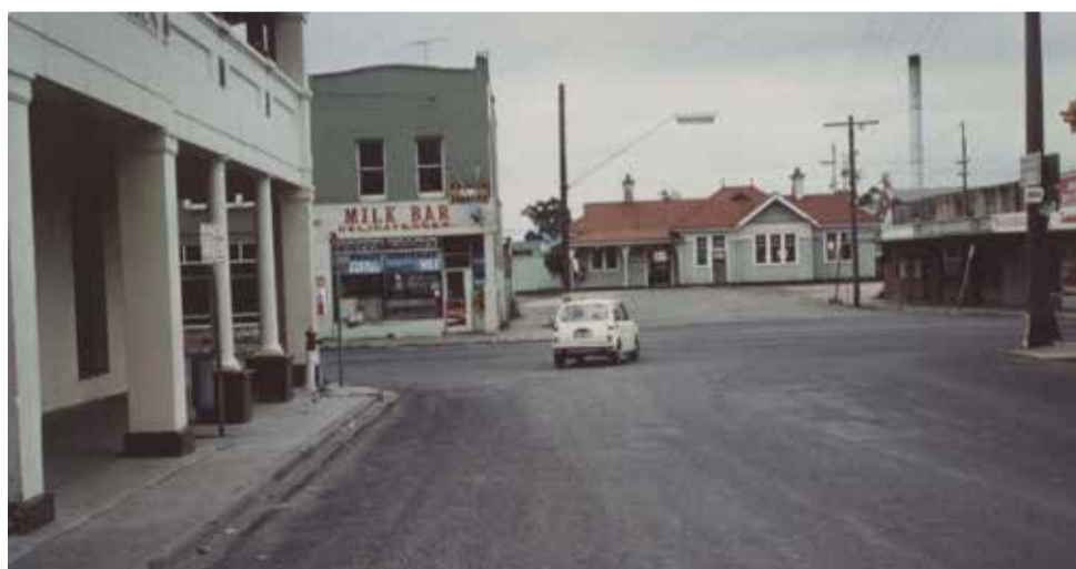
Looking south towards the railway station from Contingent Street before the duplication of the highway through Trafalgar. The shops on the south side of Main Street (now Princes Highway) were demolished to allow for the highway's duplication
