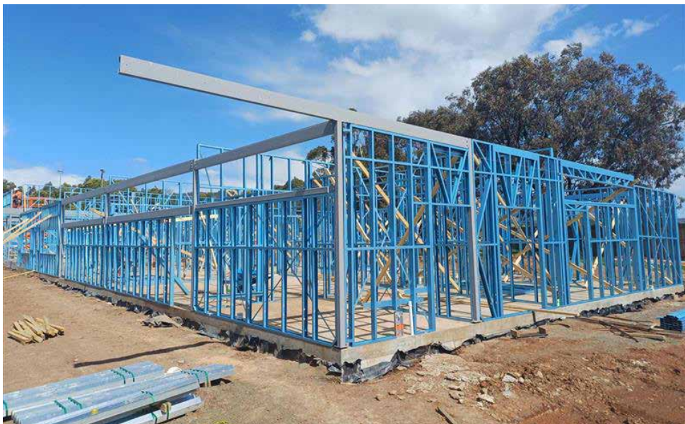
Structural steel and lightweight framing are now in place for the pavilion.
