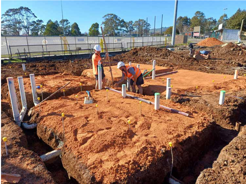
Construction is underway at Dowton Park. All images supplied.
