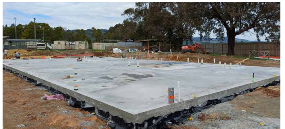
The concrete slab for the pavilion has been poured.
