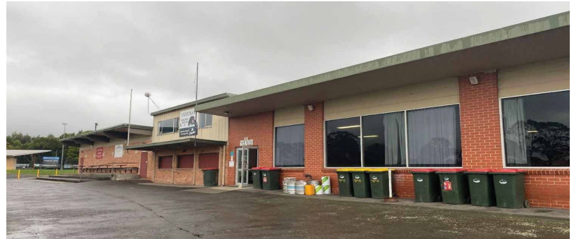
The existing pavilion at Downton Park which was built in 1988
