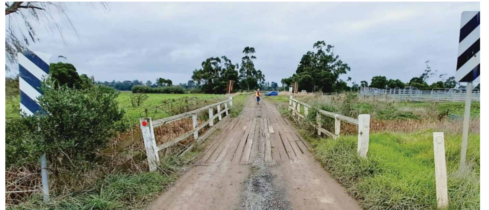
The timber bridge along Factory Road
