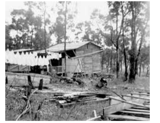
Recycled packing crates were used to build this 1950's home in Traf East.
