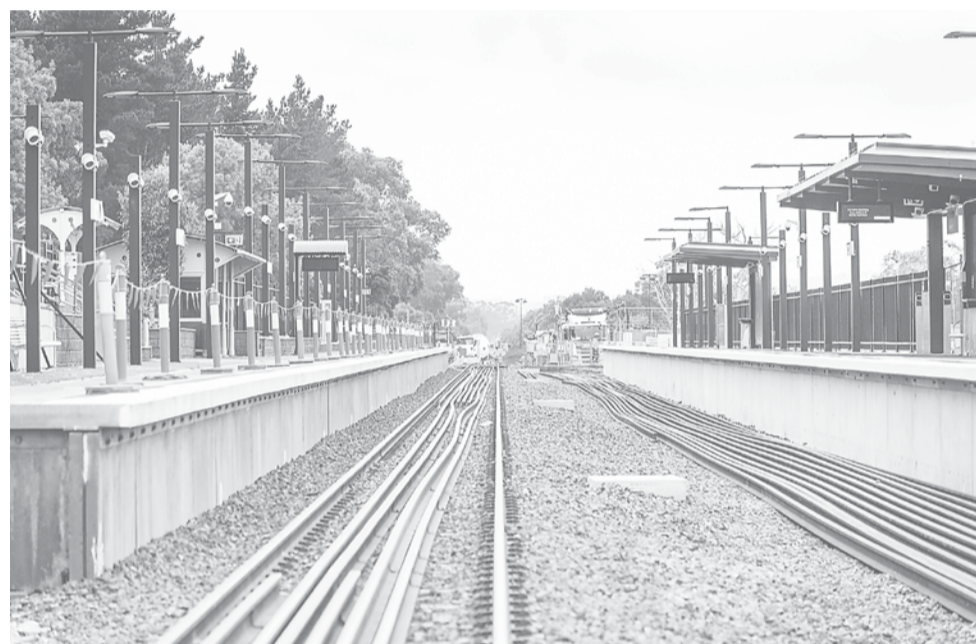
Sections of rail between the existing and new platforms at Bunyip Station before being installed as part of new, duplicated track in January.
