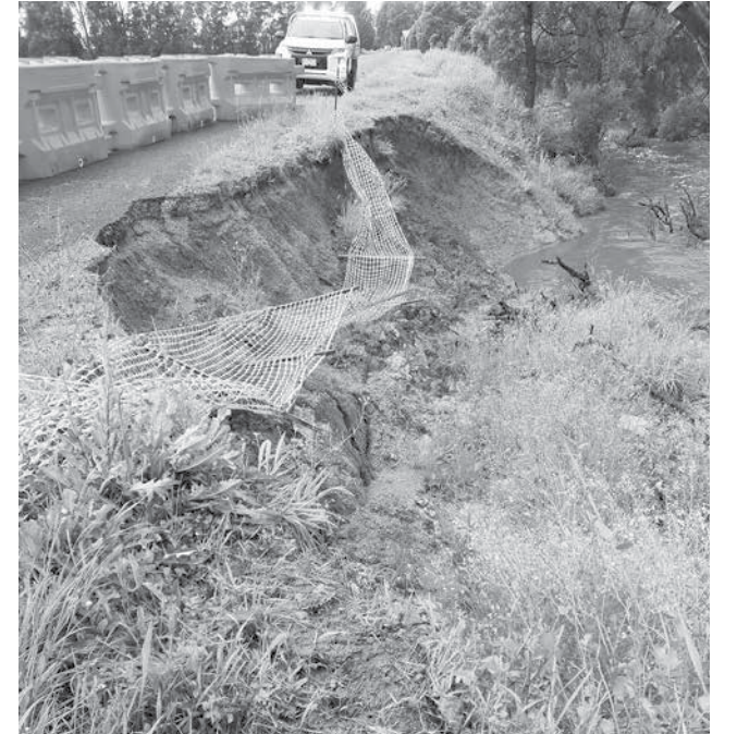
A section of the Moe Drain bank at the western end of North Canal Road that was washed away earlier this year, requiring rock stabilisation works to be undertaken to secure the road pavement
