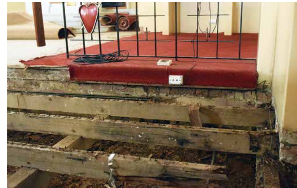
White ants totally destroyed parts of the church.
