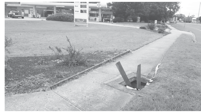
A drain lid collapsed on the footpath near the Shell Service Station
